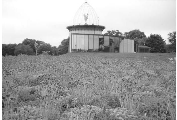
Green roof, Stepping Stones Museum for Children, Norwalk, CT.
